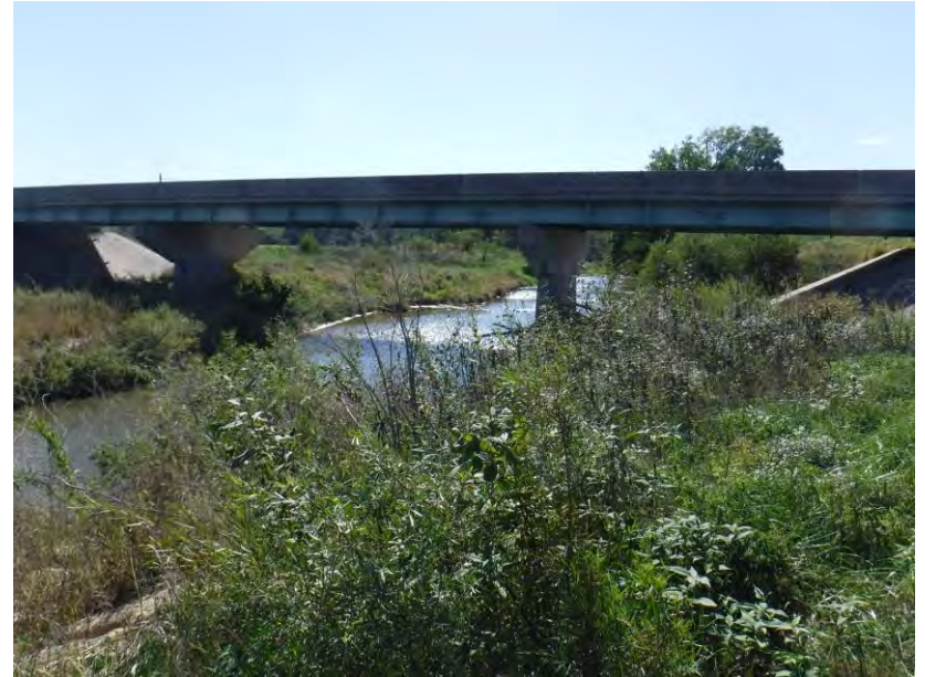
Stream US to DS, North Looking South
