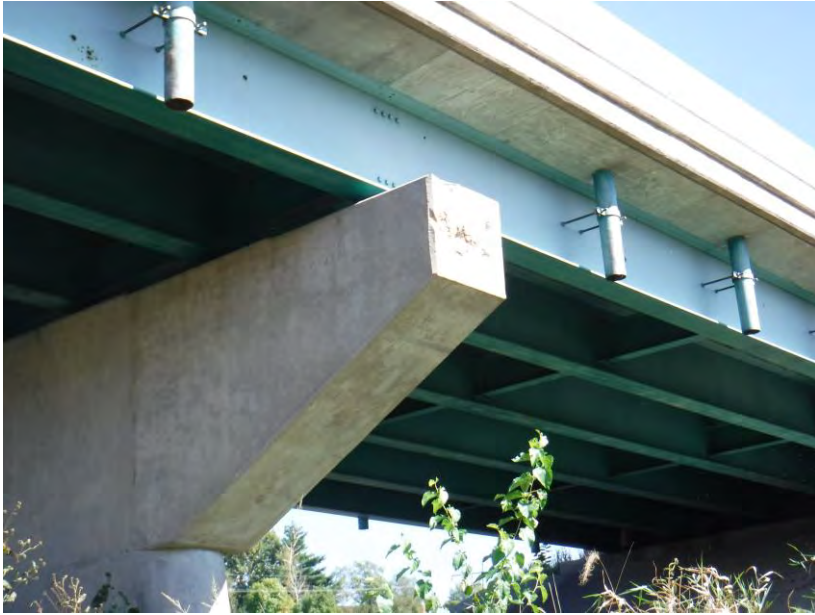
East Pier, South End
