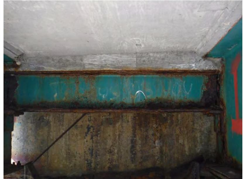
West Abutment, 1 st Diaphragm from South Edge, Hole
