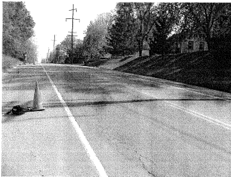
Figure 4. Sample Photograph of an Inspection Unit and Equipment Layout
