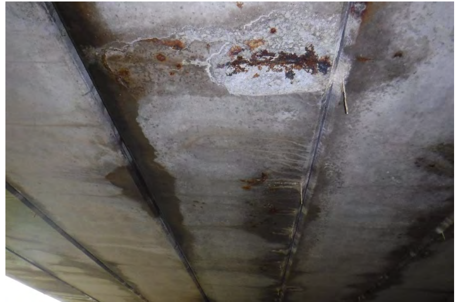
4 TH BEAM FROM NORTH EAST SPAN
