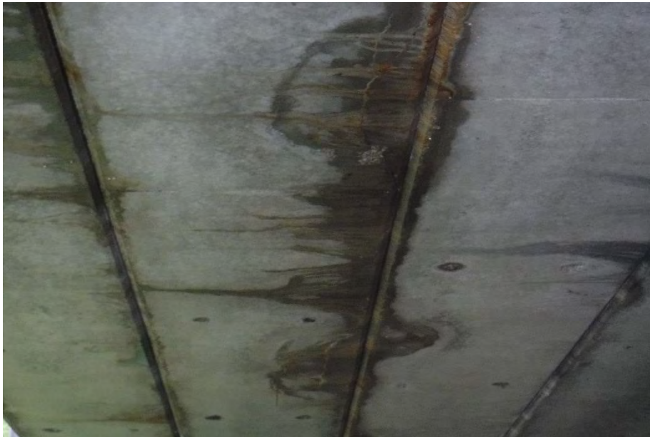
2 ND BEAM FROM SOUTH CENTER CPAN
