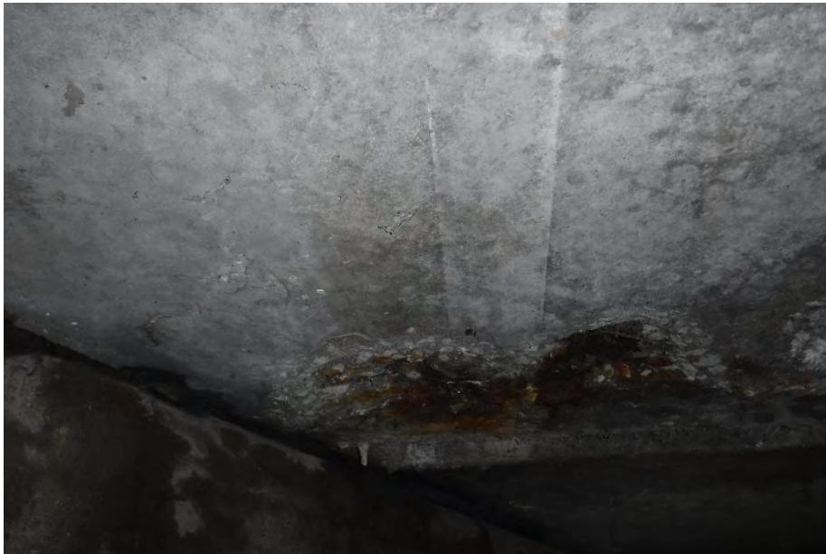
4 TH BEAM FROM NORTH WEST SPAN
