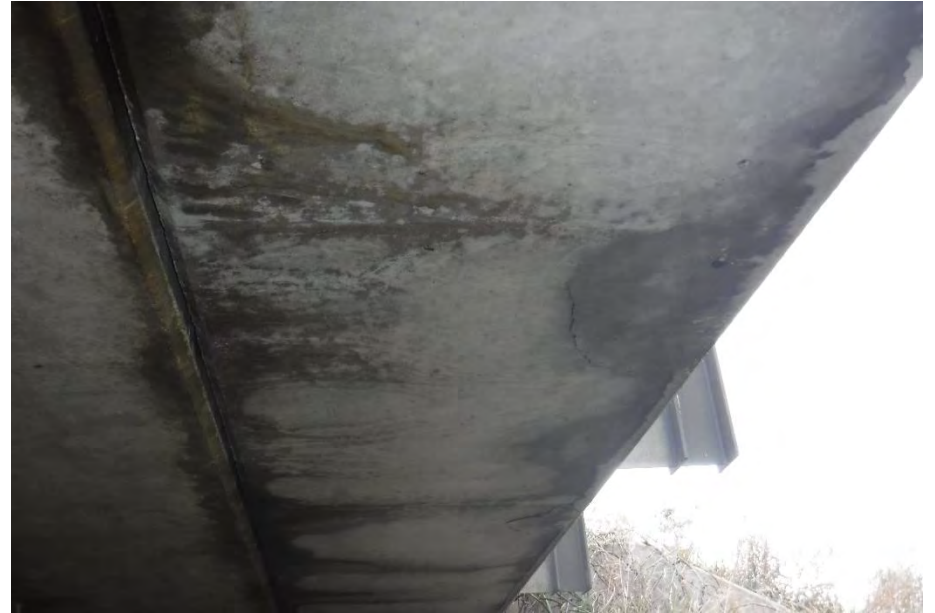
EAST SPAN SOUTH EDGE BEAM
