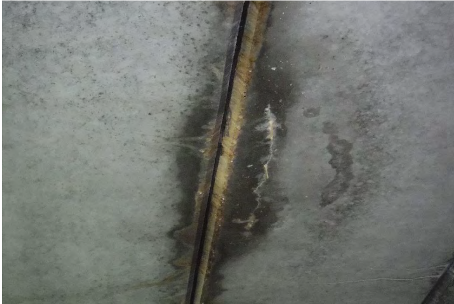
3 RD BEAM FROM SOUTH CENTER SPAN
