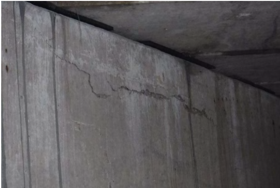
EAST SIDE OF EAST PIER CAP
