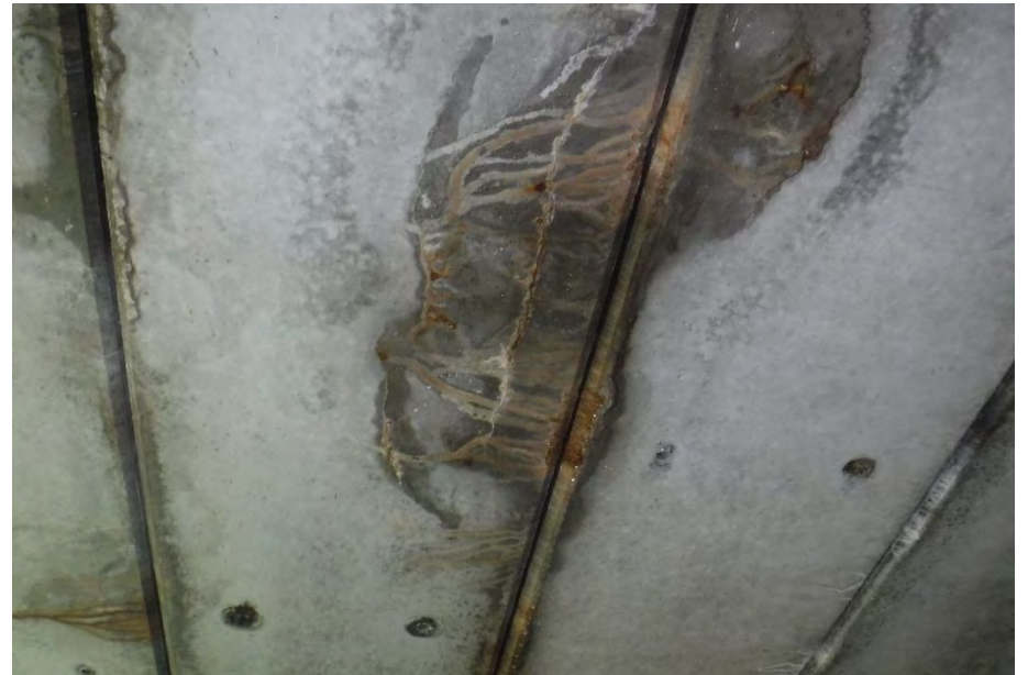
2 ND BEAM FROM SOUTH CENTER SPAN
