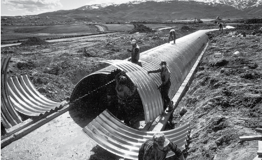
Plates are positioned by hand are ready for assembly.
