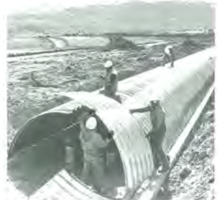
In-place structure assembly often negates the need for conventional lifting equipment.
