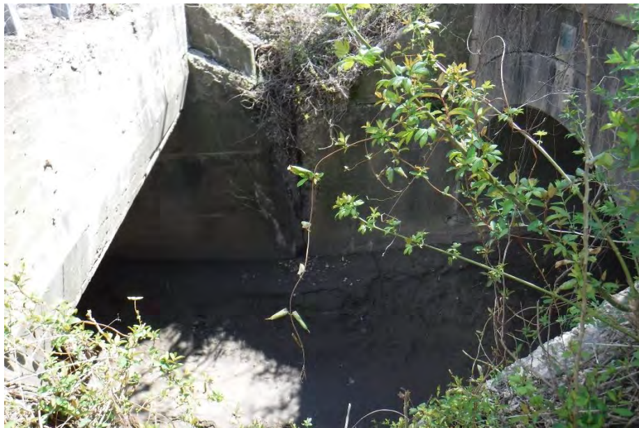
Space between 072-3095 and RxR Structure
