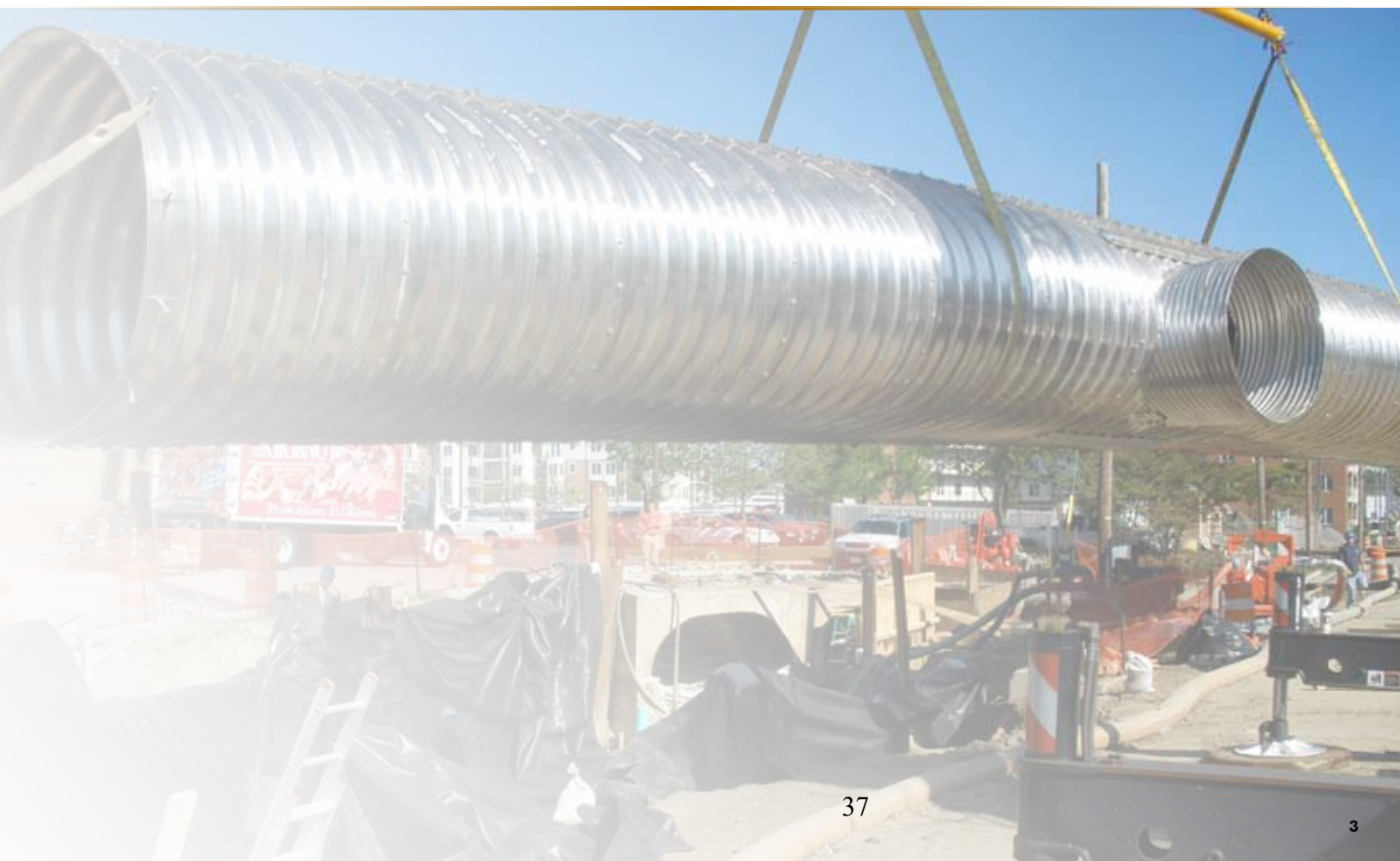
The interior of this deteriorating stone arch bridge was relined with aluminum structural plate.
