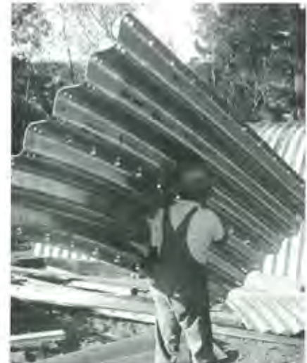
Individual plates are generally light enough to be handled by one worker.
