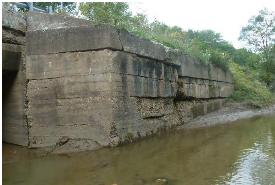
Northwest retaining wall
