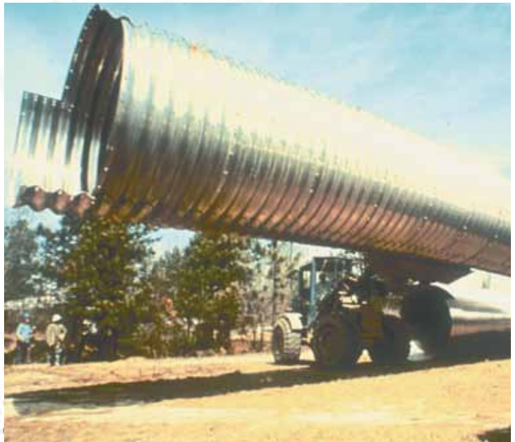
This front end loader easily handles this 50' section of round pipe.
