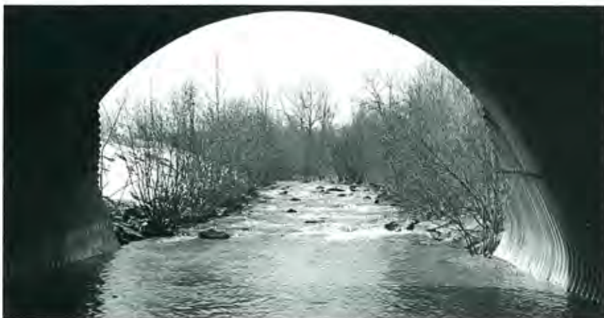
Aluminum structural plate structures offer superior corrosion resistance and many decades of maintenance-free service life.
