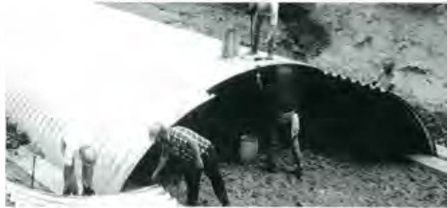
This 3-plate arch structure assembles nicely into the slotted concrete footing.
