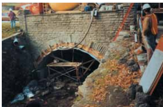
The interior of this deteriorating stone arch bridge was relined with aluminum structural plate.
