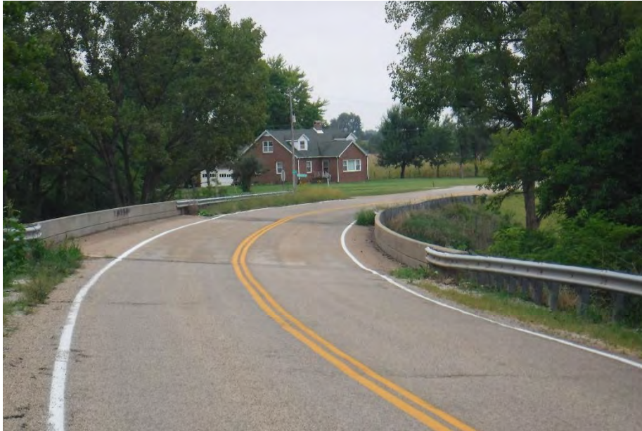
ROAD LOOKING SOUTH
