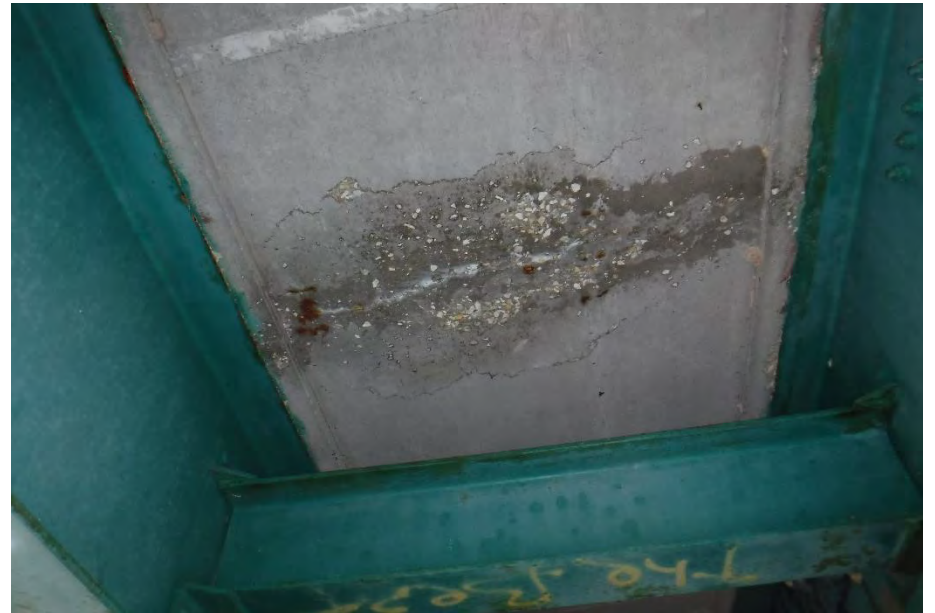
DECK NORTH SPAN
