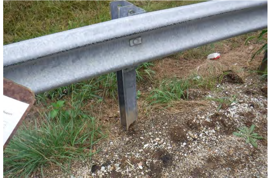
TYPICAL RAISED GUARDRAIL POST
