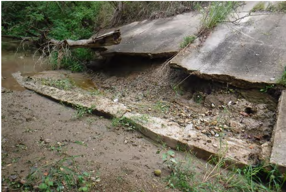
NORTH SLOPE WALL UPSTREAM
