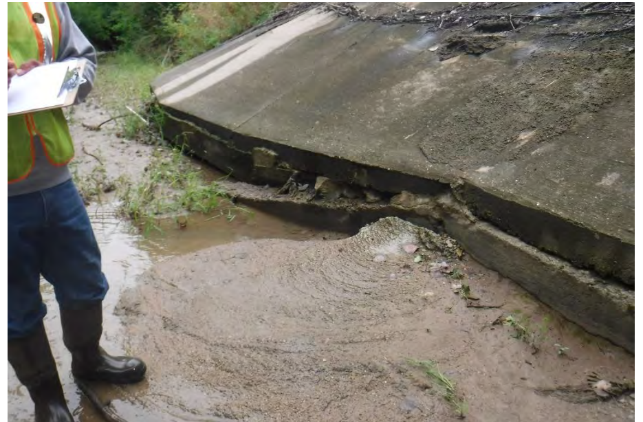
EXPOSED SOUTH SLOPE WALL TOE
