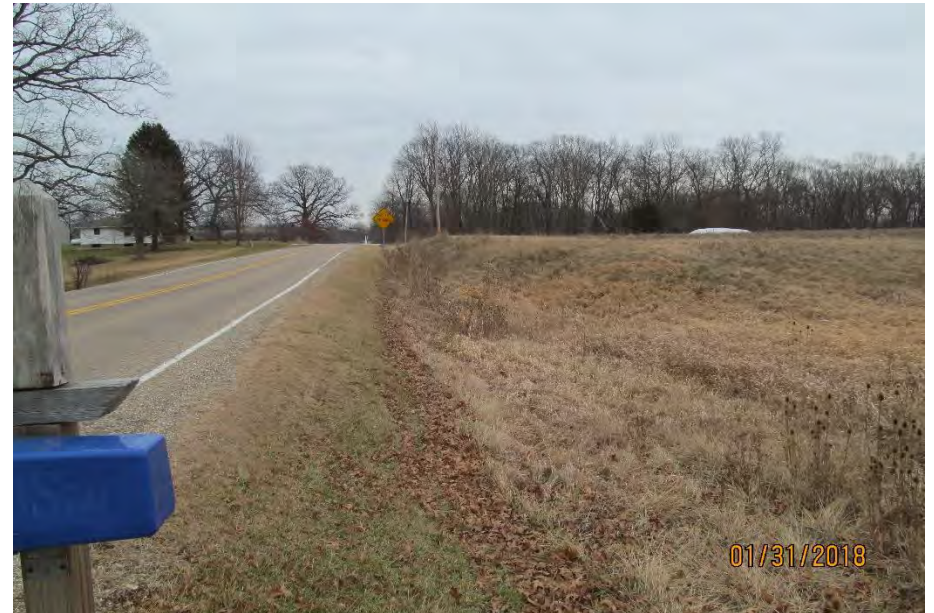
South side of road – Upstream end of culvert.
