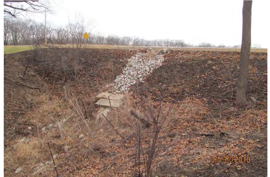
North foreslope of road.
