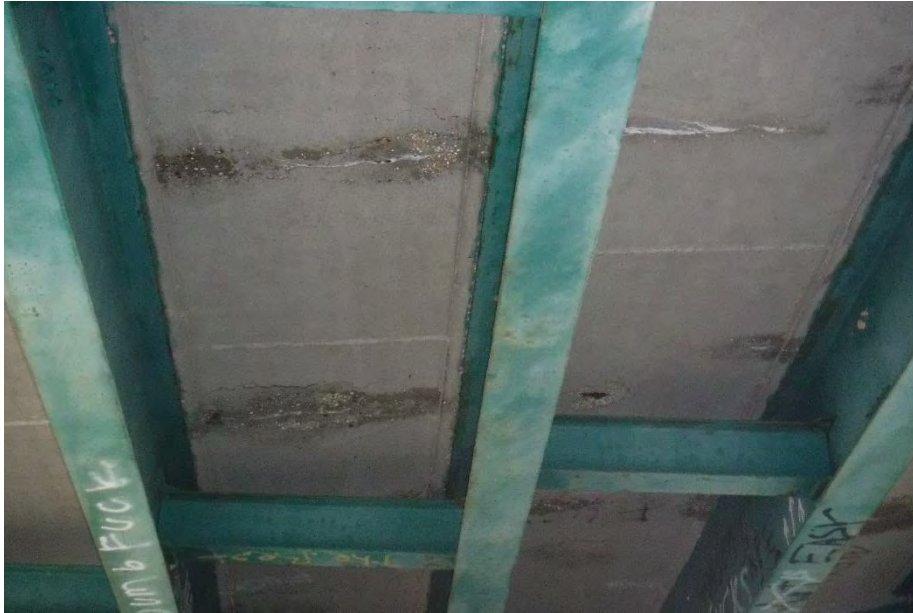
DECK NORTH SPAN
