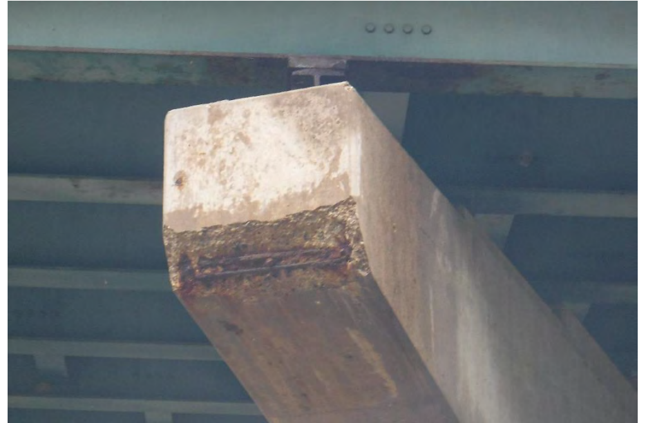
WEST EDGE NORTH PIER CAP
