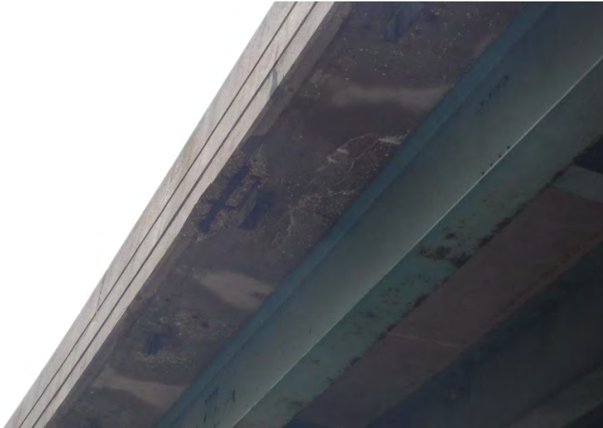
WEST EDGE AROUND DRAIN
