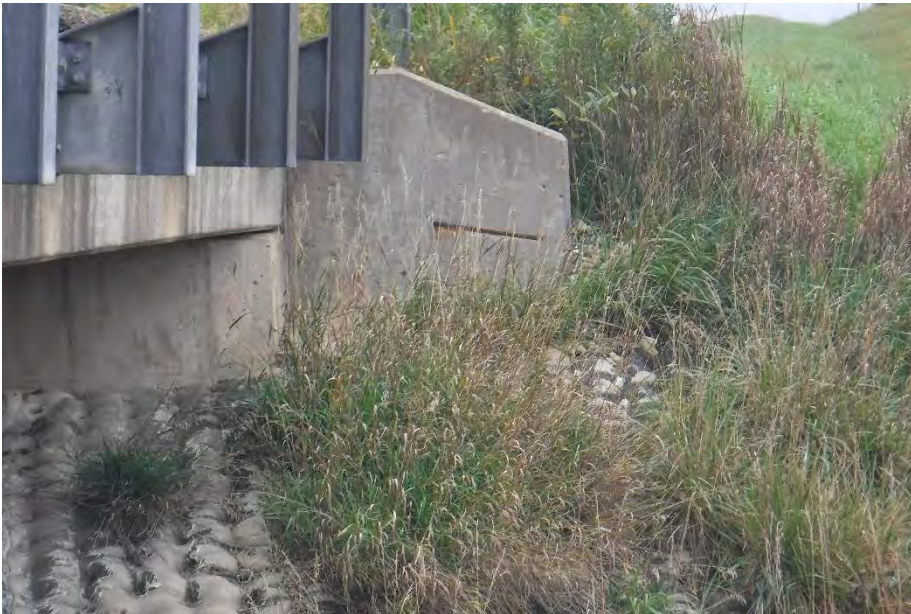
SOUTHWEST WING WALL
