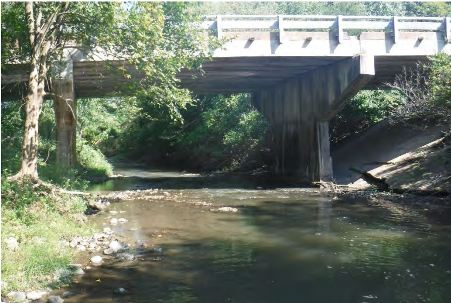
STREAM BED FACING EAST
