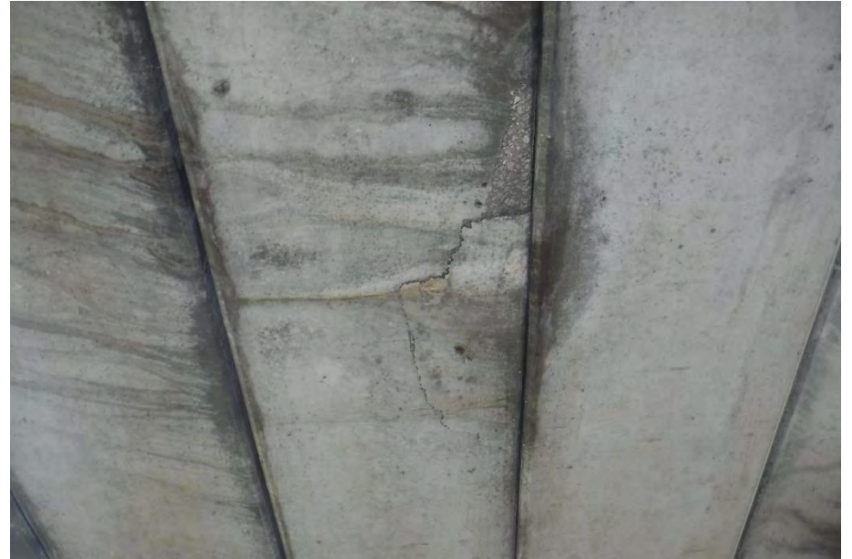
4 TH BEAM FROM EAST, CENTER OF SPAN
