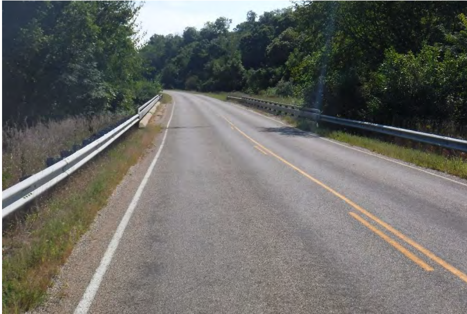
ROAD ALIGNMENT FACING SOUTH
