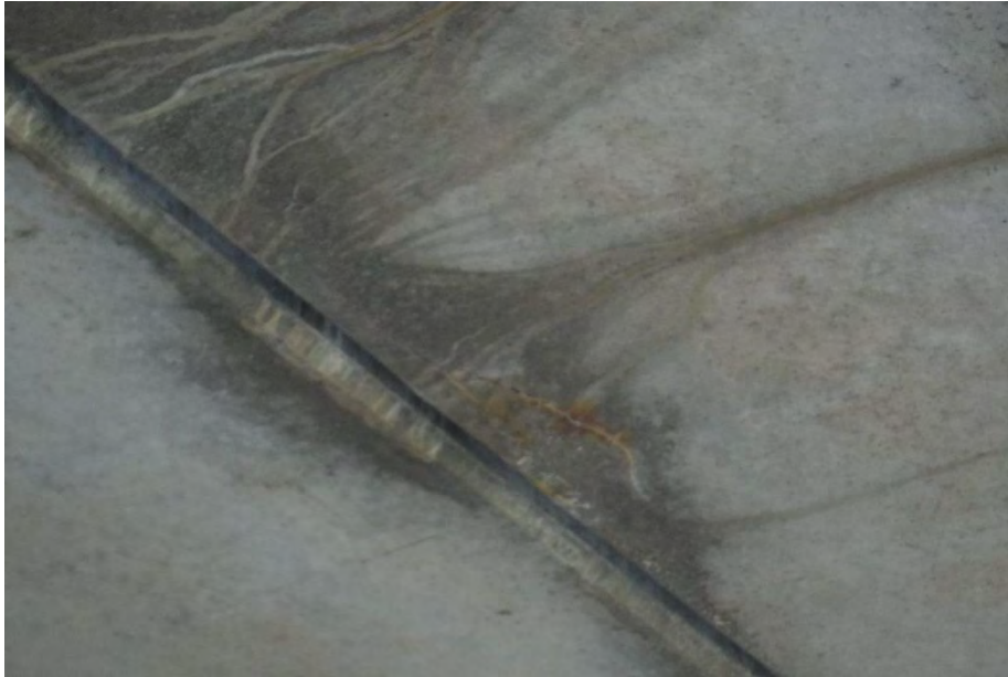
4 TH BEAM FROM WEST, SOUTH QUARTER
