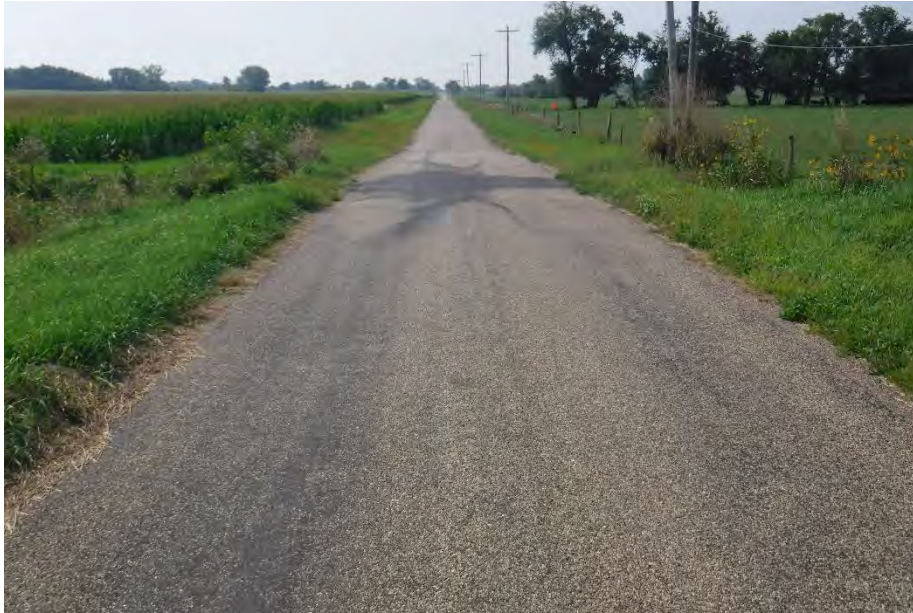
Road Looking South
