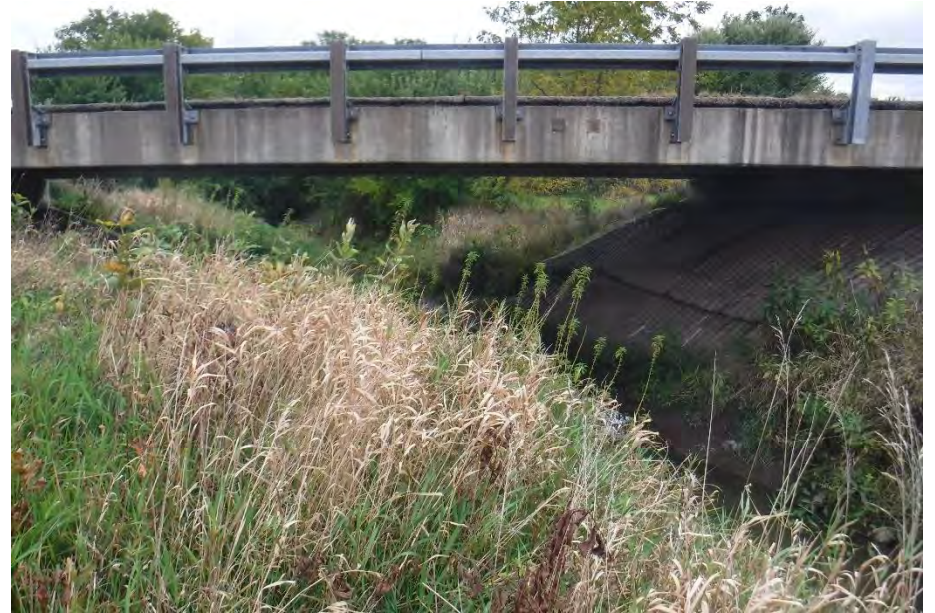
UPSTREAM LOOKING DOWNSTREAM, WEST TO EAST
