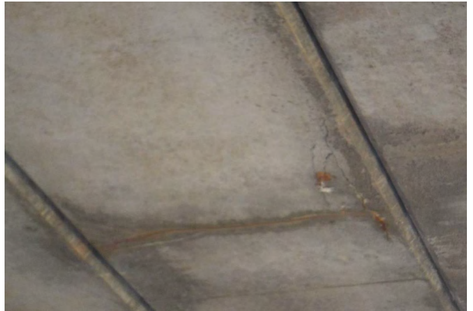
4 TH BEAM FROM WEST, SOUTH QUARTER
