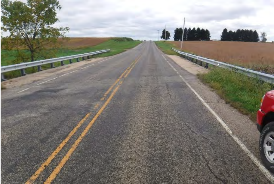
ROAD LOOKING SOUTH
